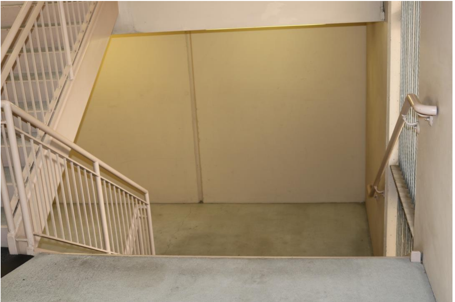
A staircase begging for a wire trap.
